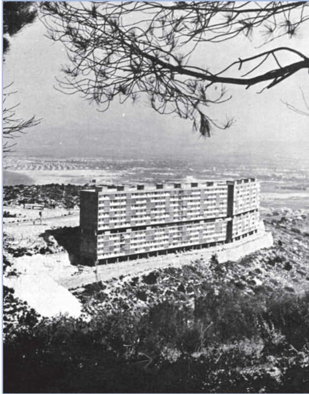
RASSCO Apartmenthaus, Ramat Hadar, Haifa, 1963 (Architekten: Al Mansfeld, Munio Gitai-Weinraub).
